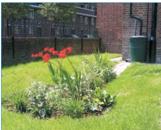
A retrofit rain garden on an Islington housing estate
