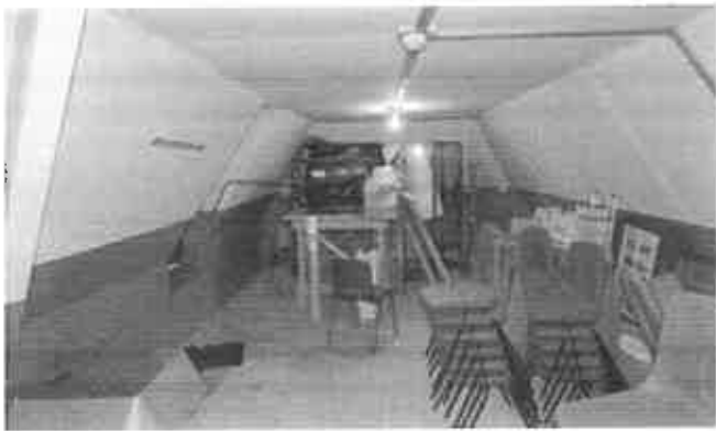
Roof void (east side)
