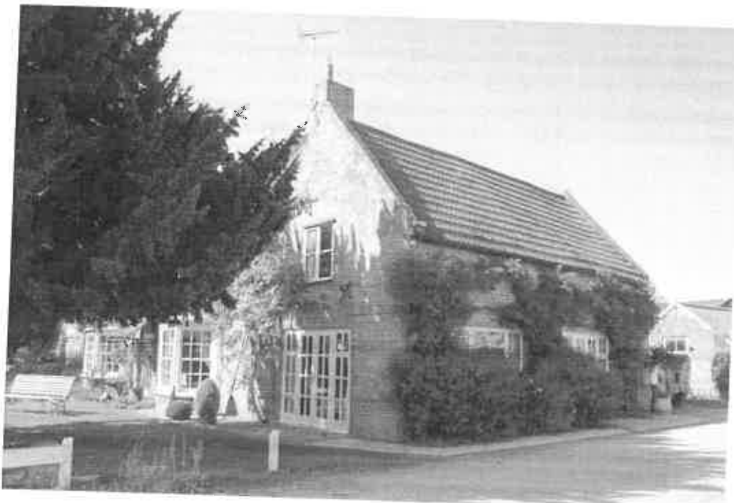
The south elevation of the south pavilion. Note the concrete tiled roof and modern fenestration.
