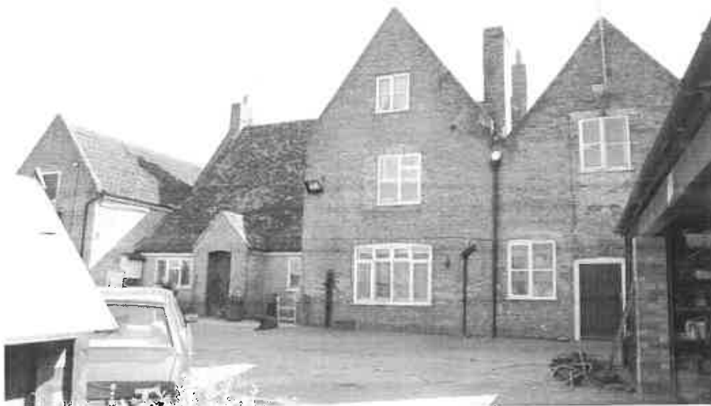
The rear elevation of Highflyer Farm showing the south range or pavilion to the left, the catslide roof of the main house, an L-shaped rear extension and the north pavilion. Note the reduced window apertures and modern fenestration.
