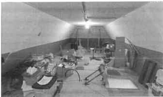
Roof void (south side)
