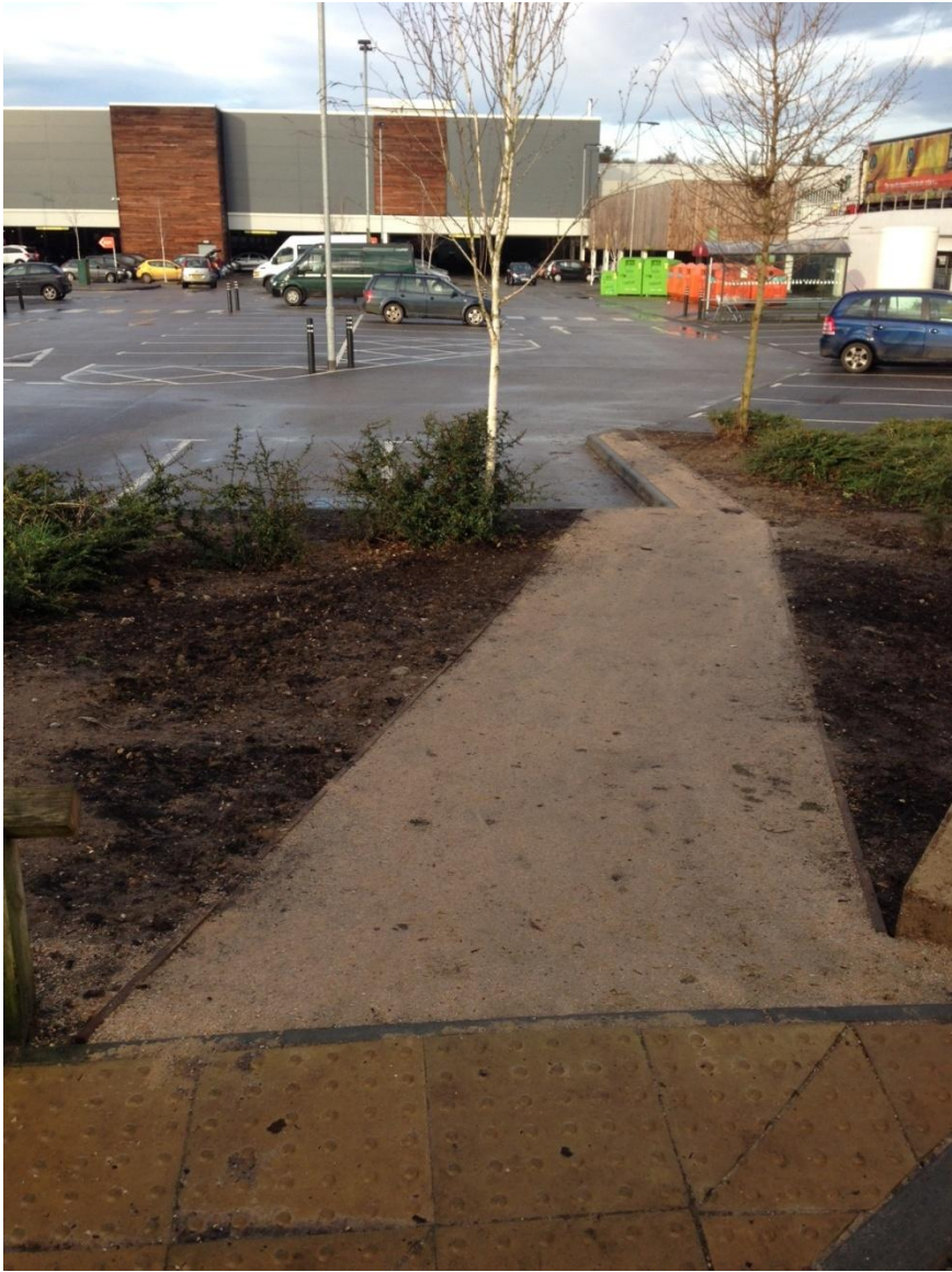
New link pathway installed by Sainsbury's
