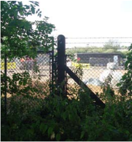
Security fencing surrounding the sewerage treatment works
