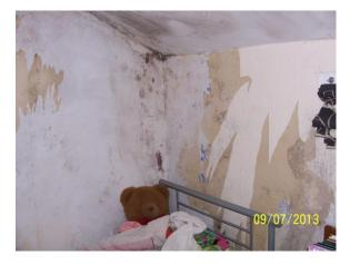
Photograph 2: Damp and mould hazard
