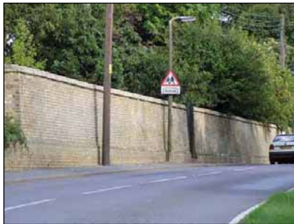
Important wall near The Green
