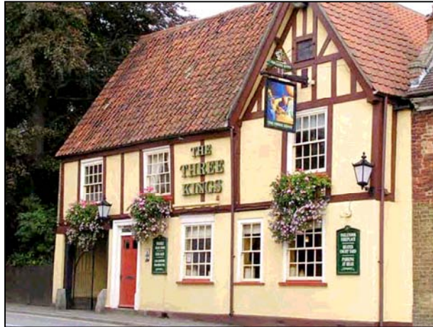
Three Kings, Station Rd
