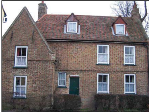
Shenstone House, North St
