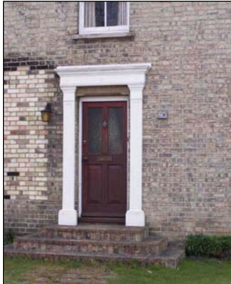
Door surround, North Street
