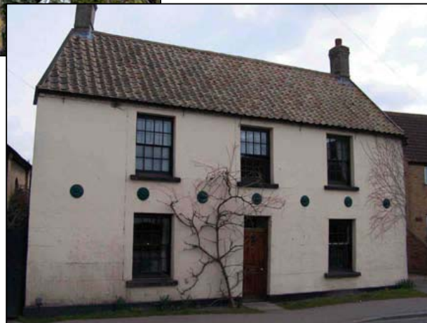
Wall tie plates to front elevation
