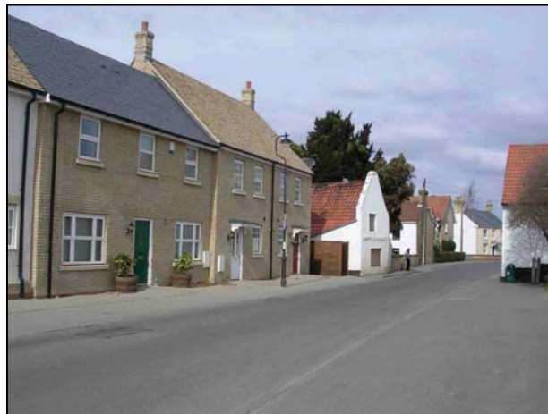
Nos.11-17 North Street
